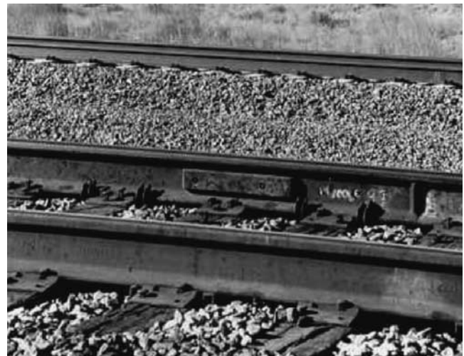
Figure 5. Elements of the strain gage protective cover.
