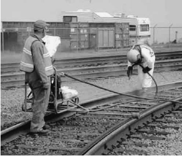
Figure 7. Sandblasting of rail prior to film coating.
