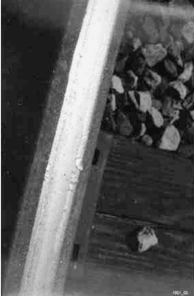
Figure 21. Top of rail flaking 4 weeks after treatment.
