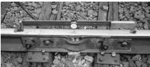
Figure 2. TCI device used for measuring differential wear of rail welds.
