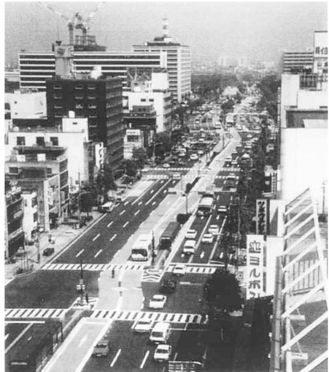
Figure 15. Key route operating on exclusive lanes in the center of the street (Nagoya, Japan).
