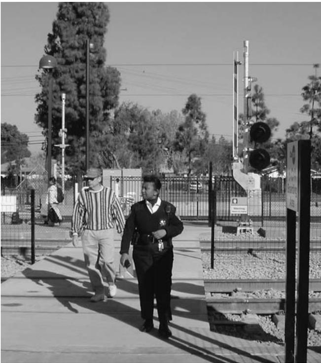
**Figure 8** Vertical Mounted Flashing Light Device with Audible.
