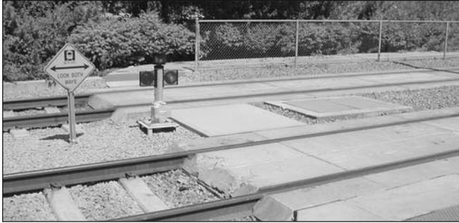
**Figure 5** Portland Tri-Met “Mini” Pedestrian Crossing Device.
