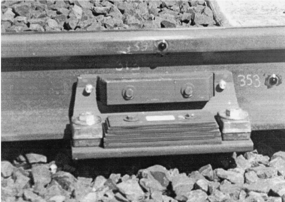
*Figure 3. Rail vibration absorber attached to 115 lb/yd RE rail at the Portland Tri-Met ballast-and-concrete-tie track.*
